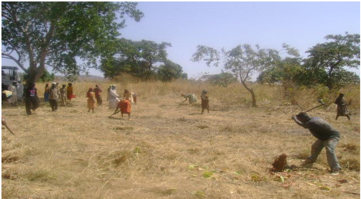
Fig 4. Communities in Dikul kebele participating in site clearing and road provision.
