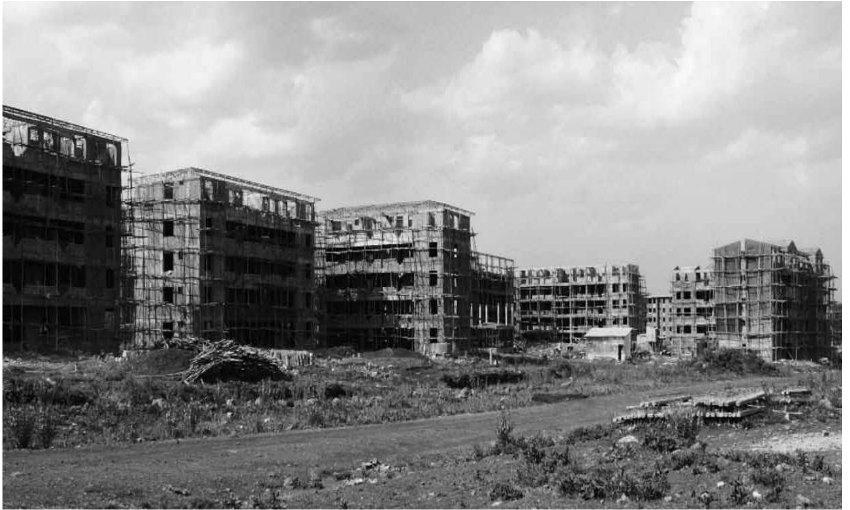
Condominium houses under construction
