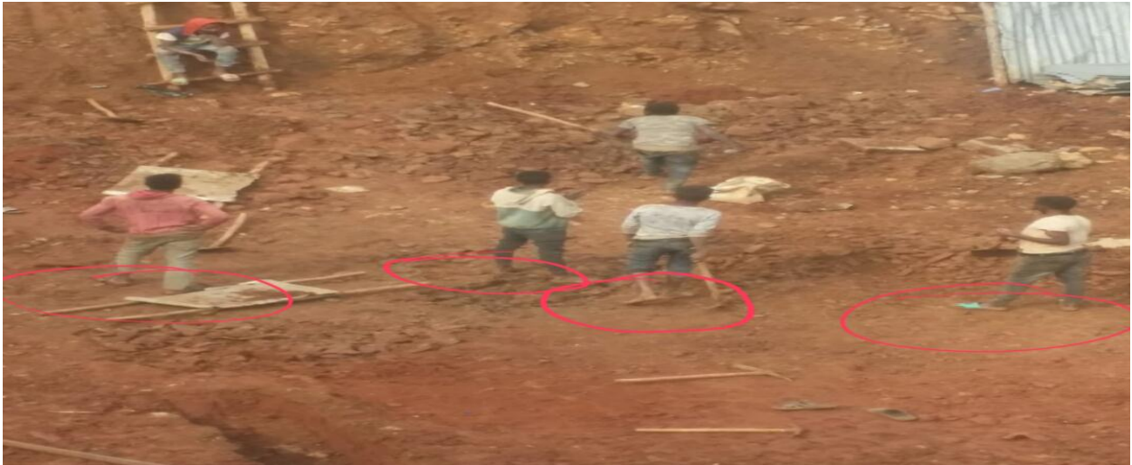
Figure 4.4 excavating without safety shoe
