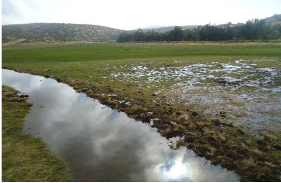
Picture 5.2. Water loss through seepage from the main canal of the scheme, Semha.
