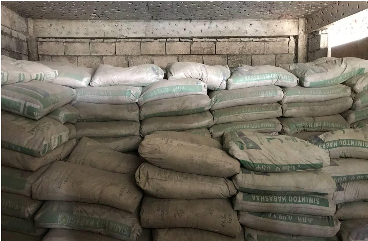
Fig: - 4.14 Recommended ways of storing cement on building site
