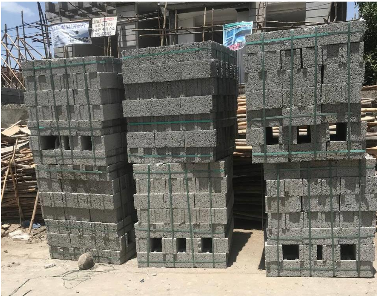
Fig: - 4.3 properly packed HCB on building construction site
