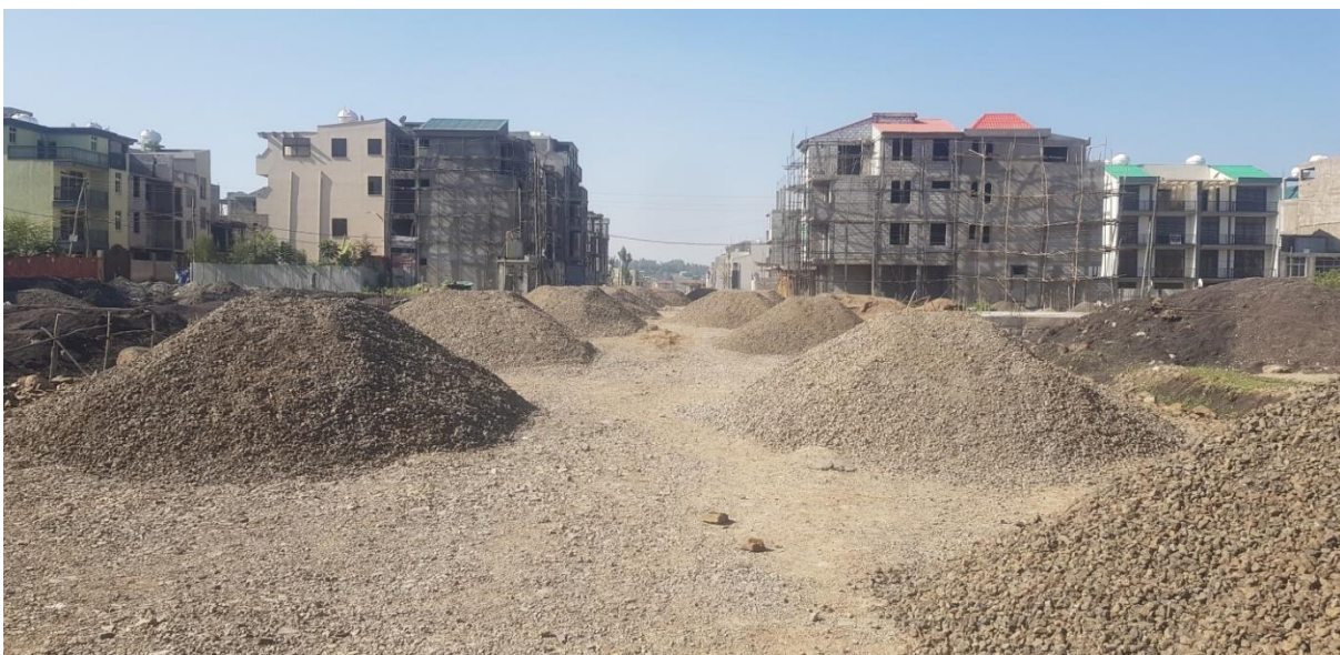
Fig: - 4.8 Good handling of sand and coarse aggregate on building site
