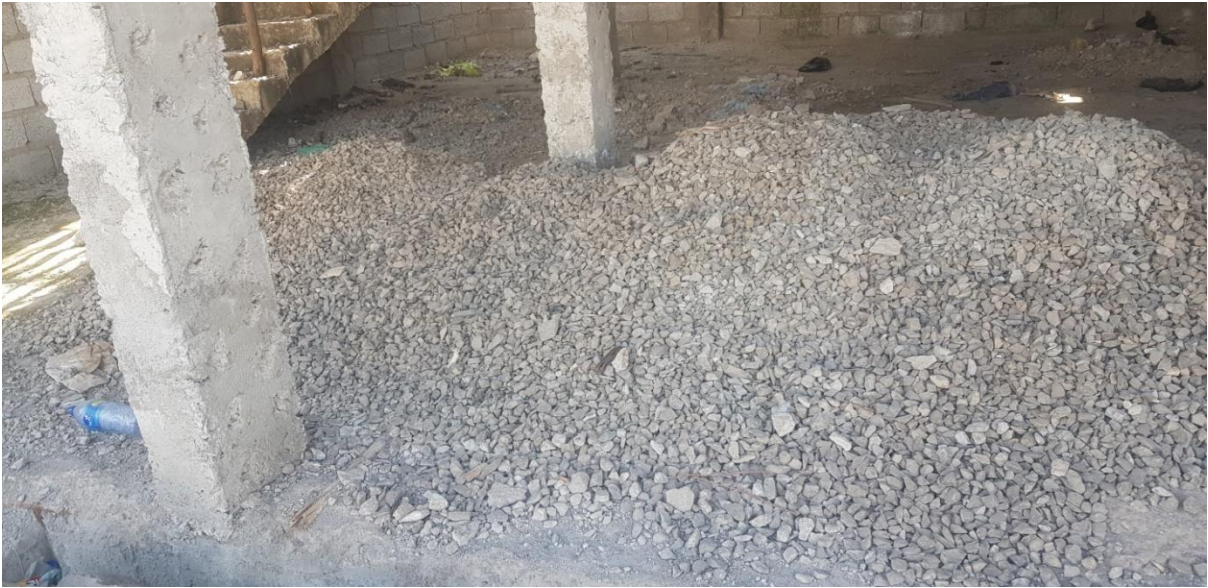
Fig: - 4.7 Poor handling of Coarse aggregate onsite
