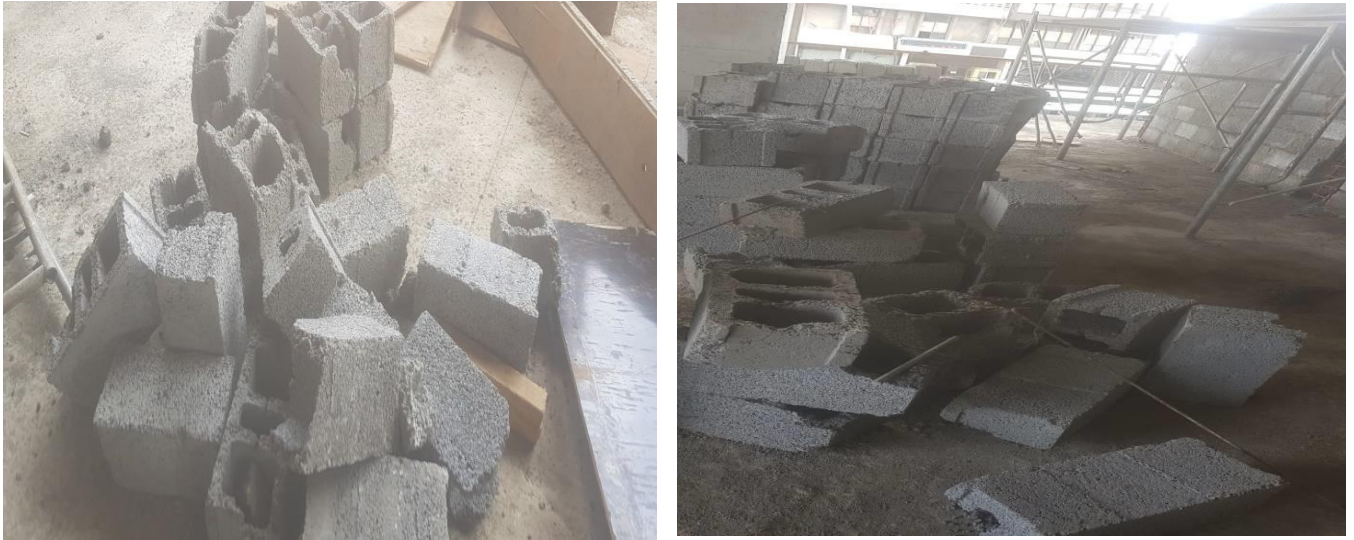
Figure: - 4.2 Wastage of HCB on building construction sites due to change orders
