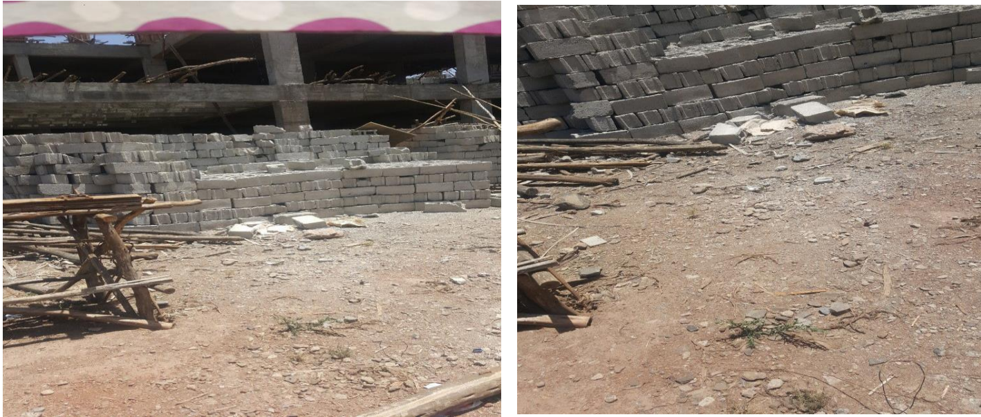
Figure 4.2 Improper storing HCB
