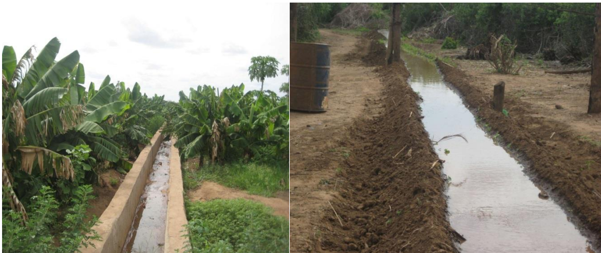
Figure 6: Concrete line and soil fenced irrigation canal at Dasheg kebele, Dolo Bay woreda
