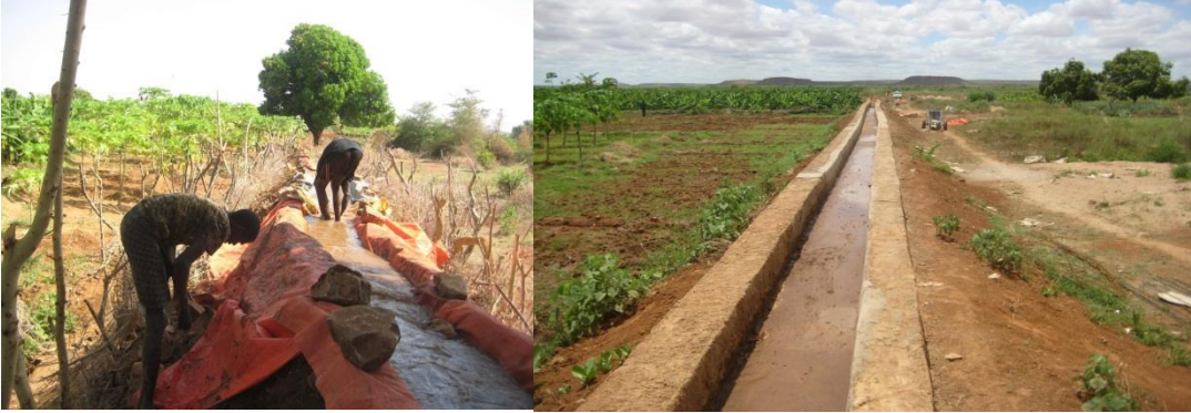
Figure 7: Soil fenced Irrigation canal while using plastic sheet at Fikow, Dolo Ado woreda
